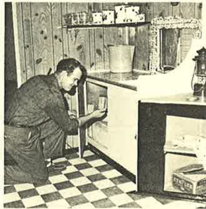
Neat, efficient mobile kitchen gets finishing touches.
