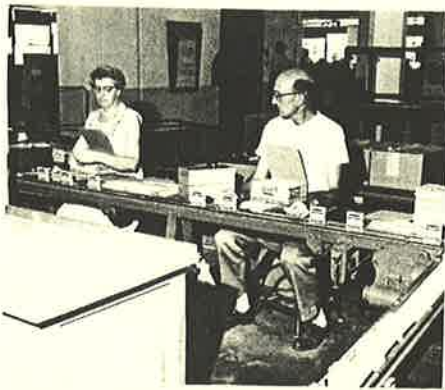
Mildred Stoller and Victor Richmond receive cartons at end of conveyor.
